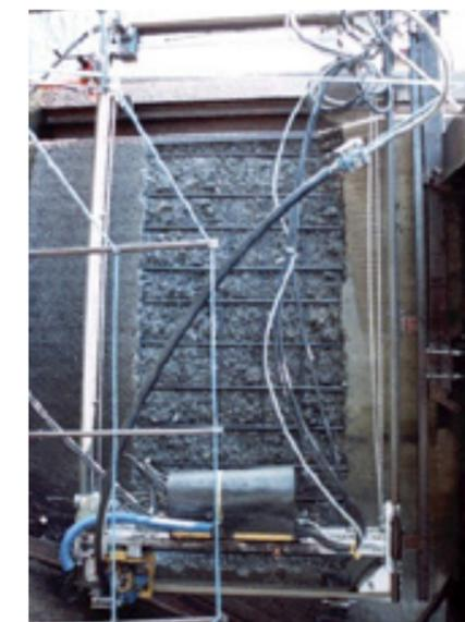
Downstream side of the dam treated by a Conjet Jetframe
