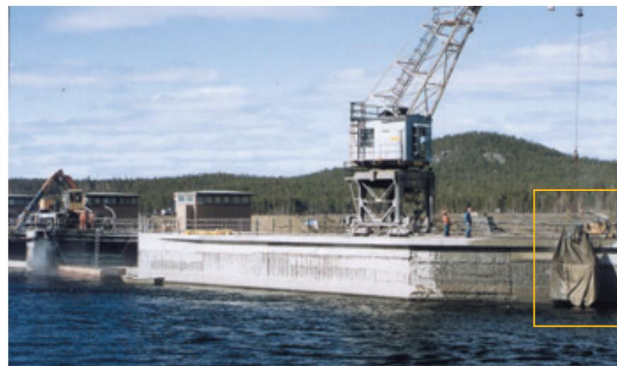
Conjet robot with vertical attachment operating from dam crest. Note debris catcher.
