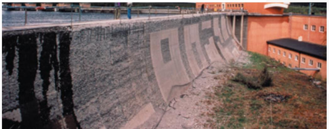
Surface at the water intake hydrodemolished down to the rebars by a Jetframe from Conjet.
