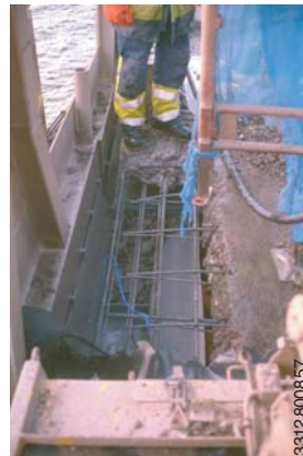
Exposed bridge deck reinforcement
