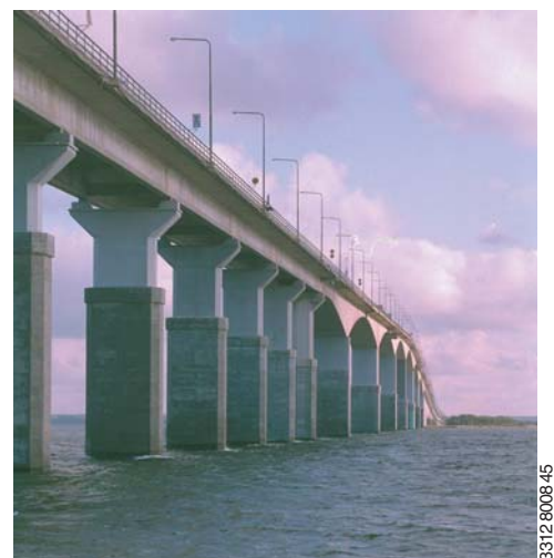
A 6 320 m long multi-span bridge.
