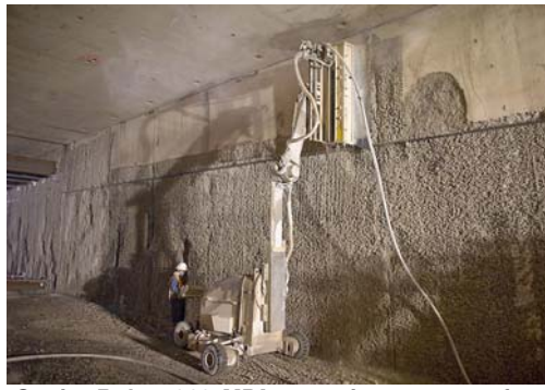
Conjet Robot 363 MPA removing concrete from the Tunnel wall
