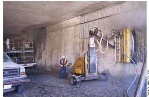
Conjet Robot 363 MPA and Conjet Robot 322 on a scaffold in the background removing concrete from the tunnel wall.
