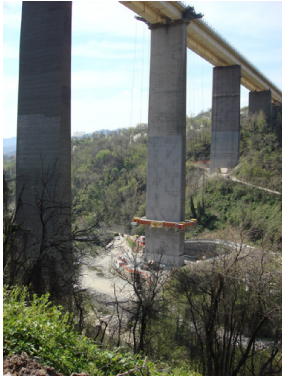
The Rio Verde viaduct is one of the tallest in Europe supported on piers up to 136m high and carries the dual two lane A15/E33 Autostrada della Cisa over a steep sided valley in the municipality of Pontremoli.
