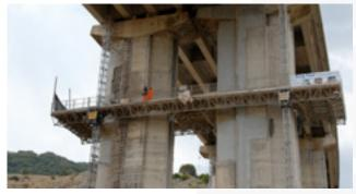
Conjet AB advised CPL to use a platform from SAFI that permitted the light flexible Conjet Robot 322 with a weight of just over one ton to operate on the platform with space enough to operate inside the lifting towers of the platform. Further was the same platform used when the concrete were replaced.
