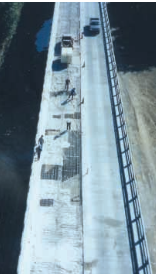
Picture shows Class III, full deck removal, made by Conjet equipment.
