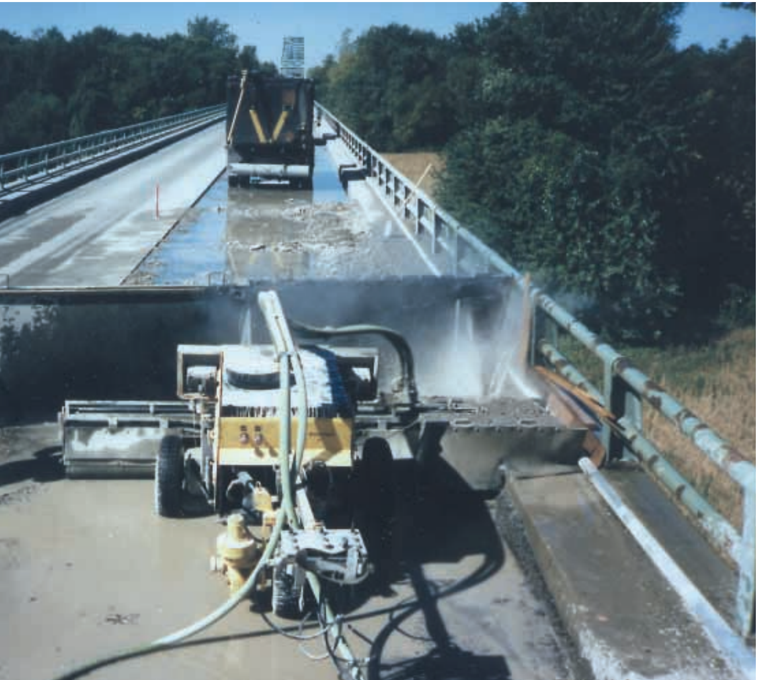
Above the Conjet Robot in full action equipped with 13 ft (3,9 m) width.
