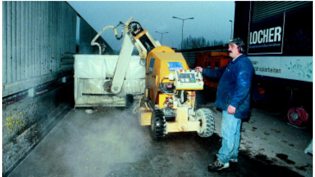
The Conjet 363 with the specially designed acoustic shroud.
