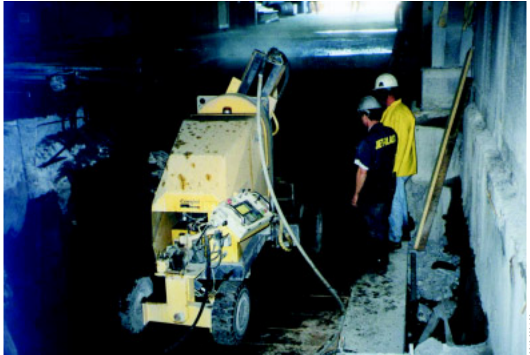
The Conjet Robot 362 in position to start the repair.
