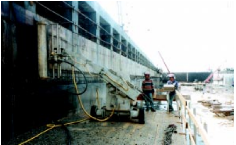
Strips of damaged concrete was removed from the dock walls.
