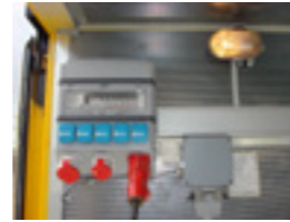
The Powerpack has an electrical distribution central, handling all electricity in the unit
